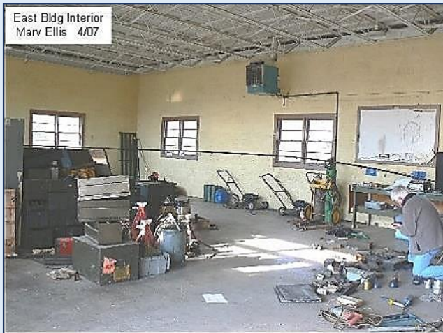
East Building Interior
