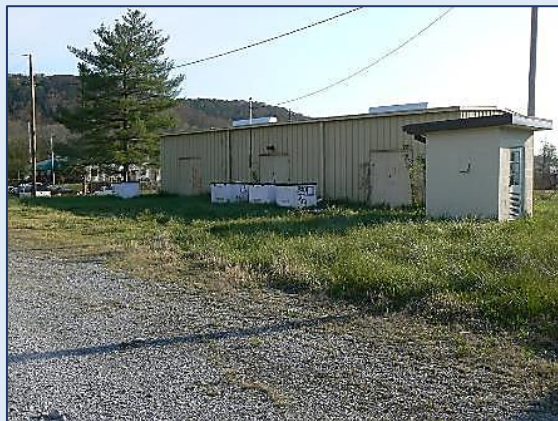
Steel Building Exterior
